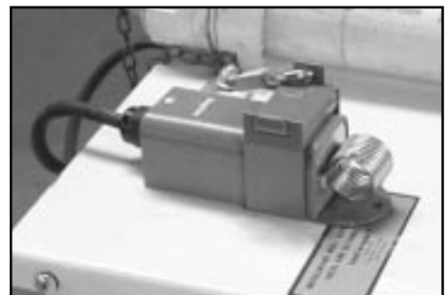
THERMOSTAT LOCK BOXES
